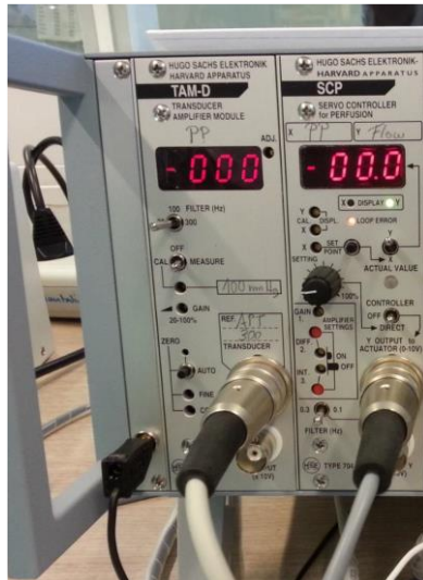
Example 1: TAM-D and SCP installed in a PLUGSYS housing Type 601
